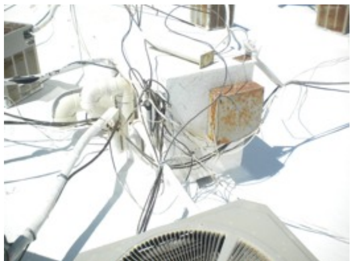
Roof of building C with new sealador
