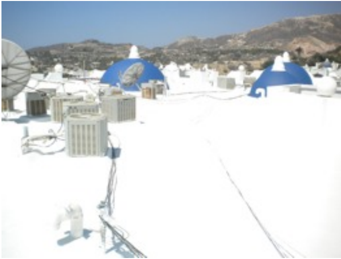
finished roof top of building c
